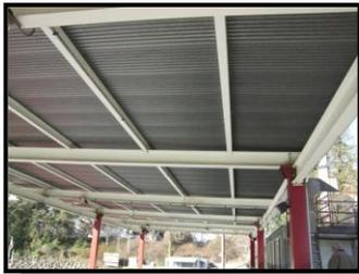
PSM acted as prime consultant for this project, which included new catwalks and roofing. When defects from original construction were discovered in the steel moment frame supporting the grandstand, we also prepared repair drawings, and observed construction.
