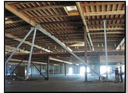
building was upgraded to resist future seismic events. Difficult geotechnical conditions (liquefiable soils) added to the complexity of this project. Additional structure (mezzanines) was added in the interior of the facility for new functions.
