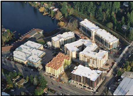
Design of a multi-building complex. Multiple framing levels over post-tensioned slabs and parking.
